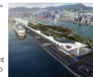
Above: The Kai Tak Cruise Terminal Building will be completed in 2013.
