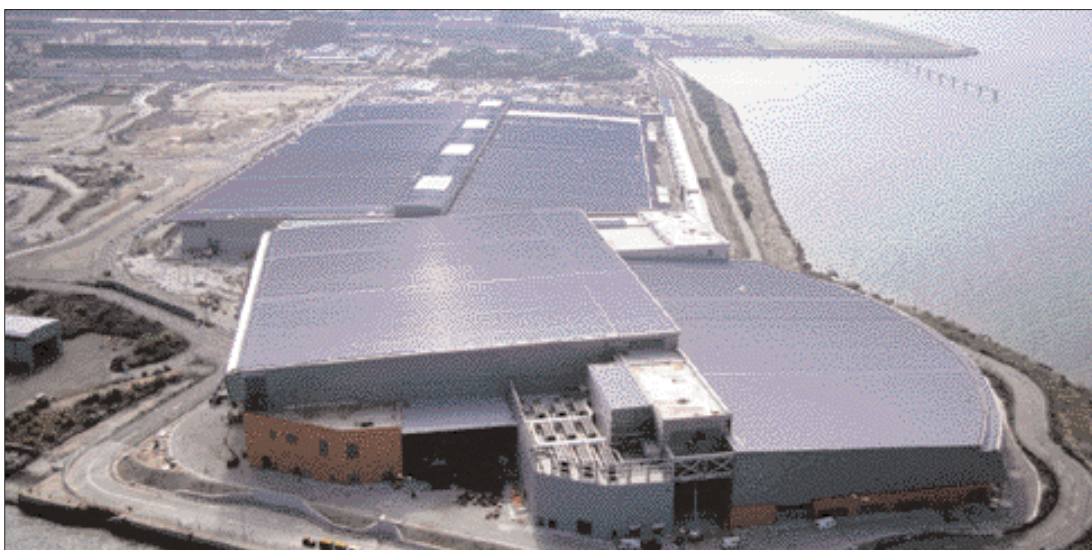
Aerial view of the AsiaWorld-Expo site on Hong Kong's Lantau Island
